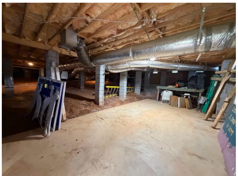
The College Hunks were a HUGE help in cleaning out the basement.
